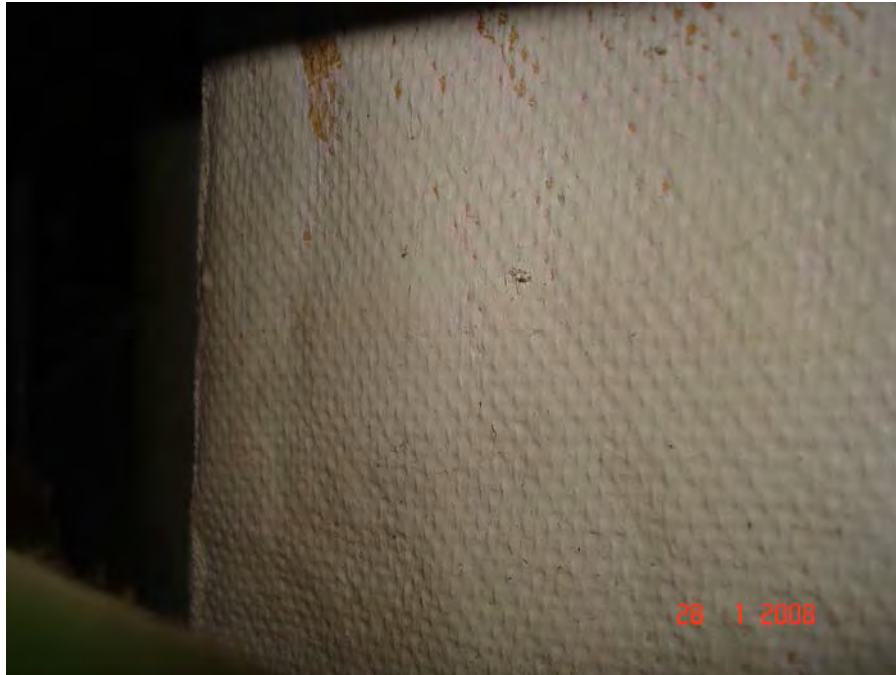
Photograph 7: View of asbestos-containing mechanical air duct insulation identified in the basement, hallway 279C (OHE Sample MA1014-37).
