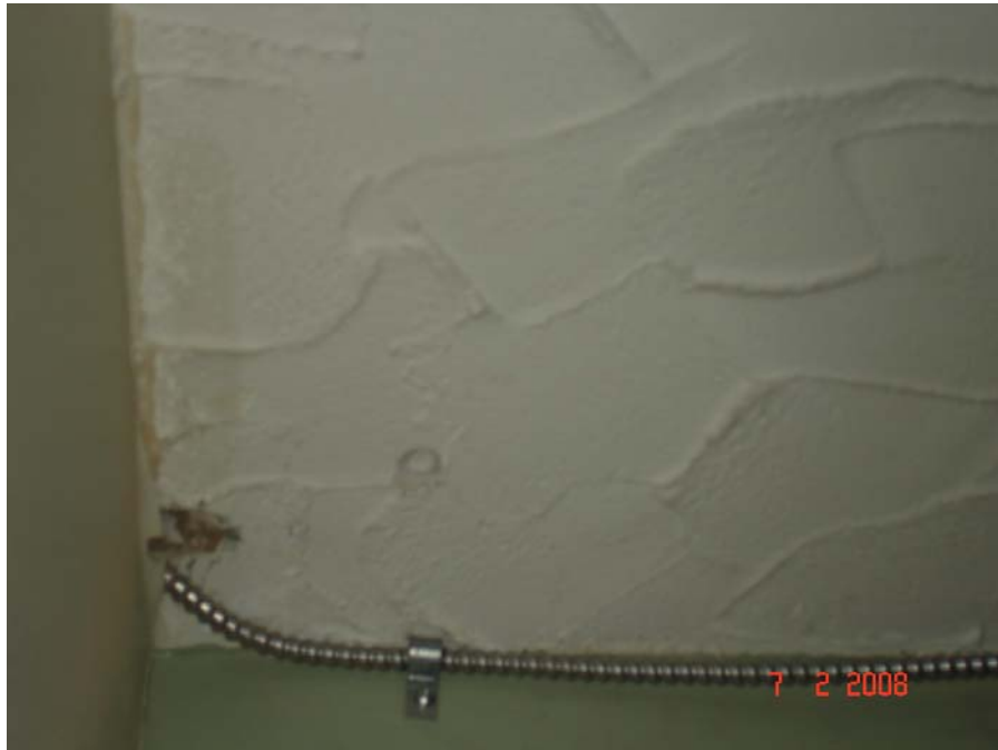
Photograph 10: View of asbestos-containing texture coat on ceiling identified on the main floor, hallway 1108 (OHE Sample MA1014-43A).
