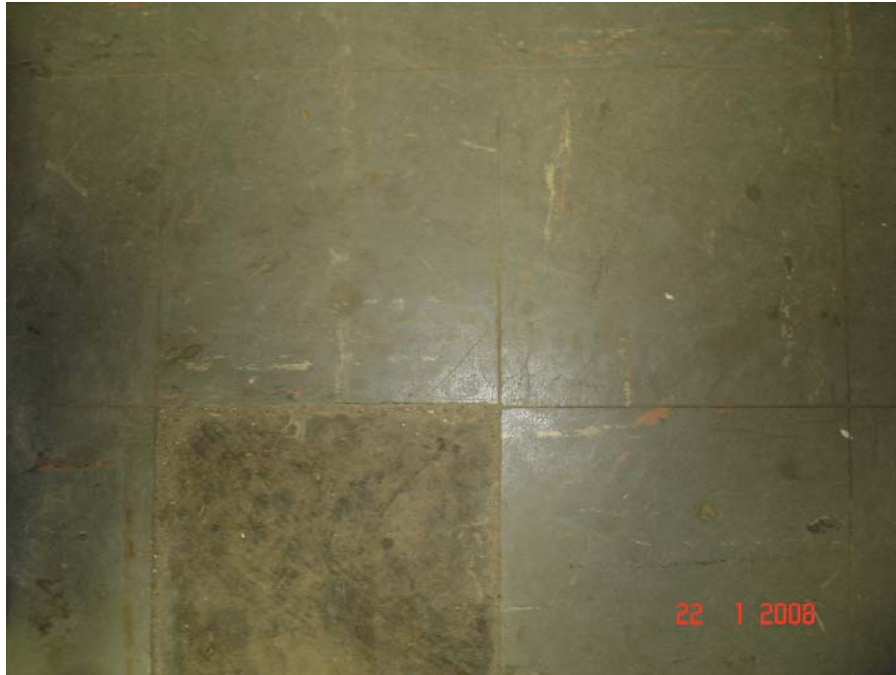
Photograph 5: View of asbestos-containing floor tile identified in the basement, Room 305 (OHE Sample MA1014-28A).
