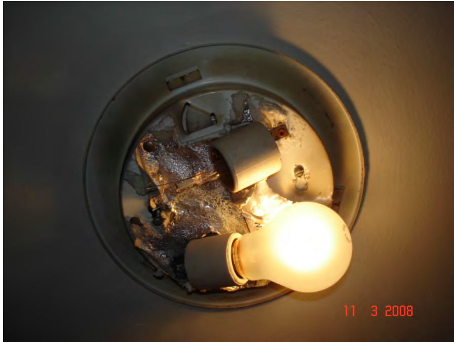
Photograph 9: View of asbestos-containing heat shield on an incandescent light fixture identified on the fourth floor, room 4014 (OHE Sample MA1014-51).
