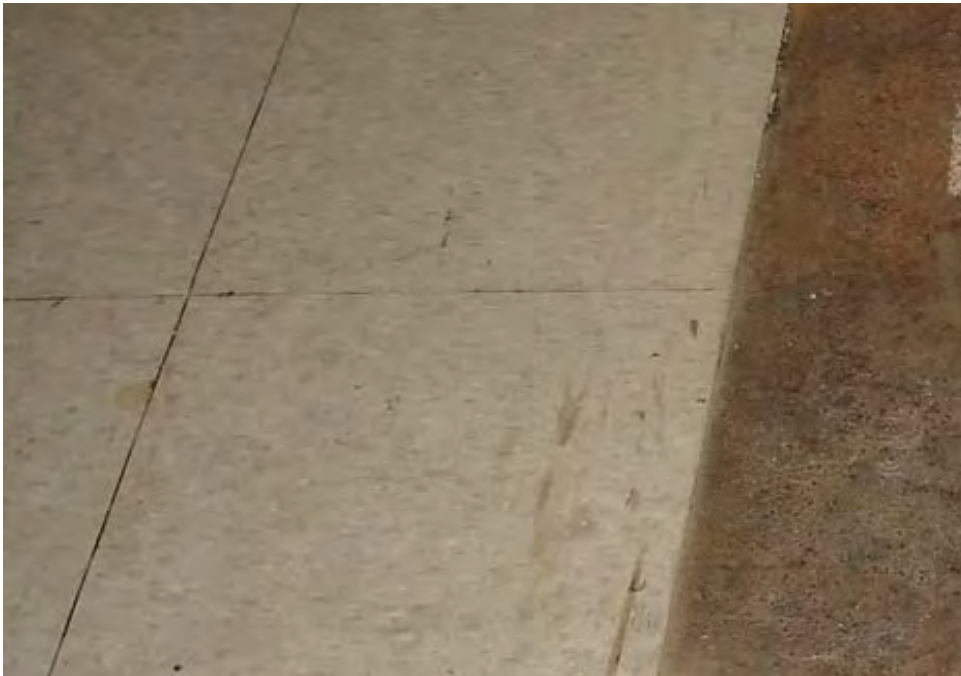
Photograph 2: View of additional type of asbestos-containing floor tile identified in the basement, hallway B113 (OHE Sample MA1014-26B).
