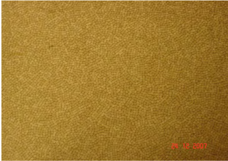
Photograph 3: View of asbestos-containing vinyl sheet flooring identified on the Main floor, room 1657A (OHE Sample MA1014-2A).
