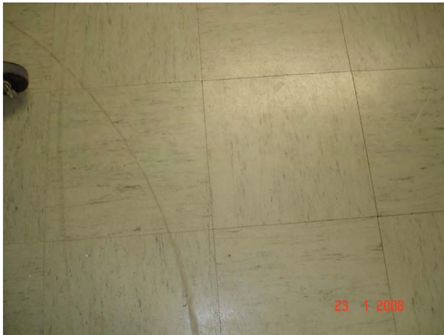
Photograph 6: View of asbestos-containing floor tile identified in the basement, room 338 (OHE Sample MA1014-30A).
